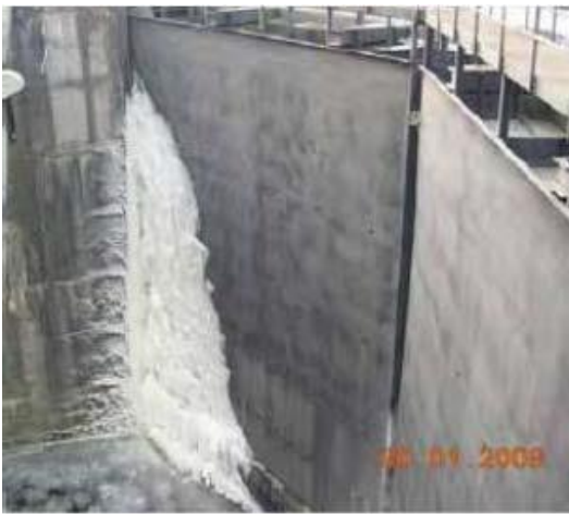
Figure 14 - Presence of ice in locks under the navigation conditions (Source: via Donau)
