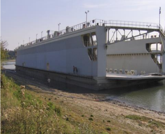
Figure 12 - Accident caused by the low level of water in summer (Source: IMST)
