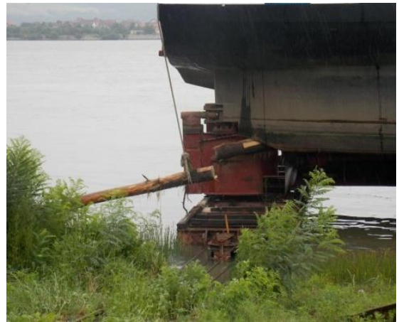
Figure 13 - Accident caused by the high level of water after flood (Source: IMST)
