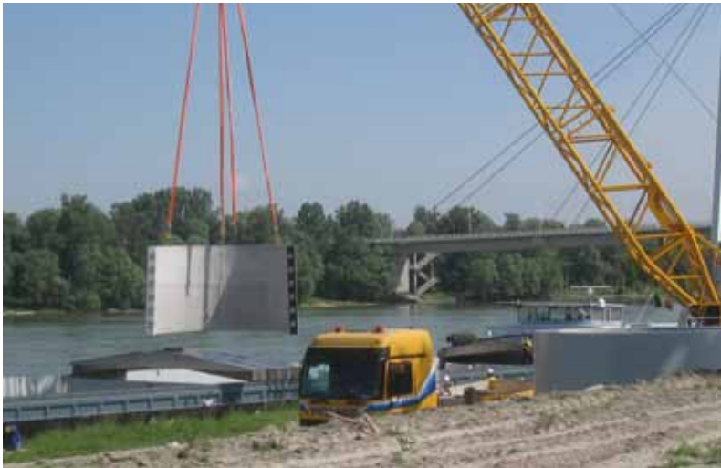
Transshipment of concrete sections in Bad Deutsch-Altenburg
