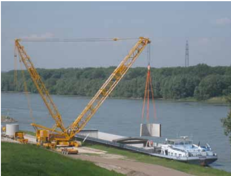
Mobile crane with caterpillar track system
