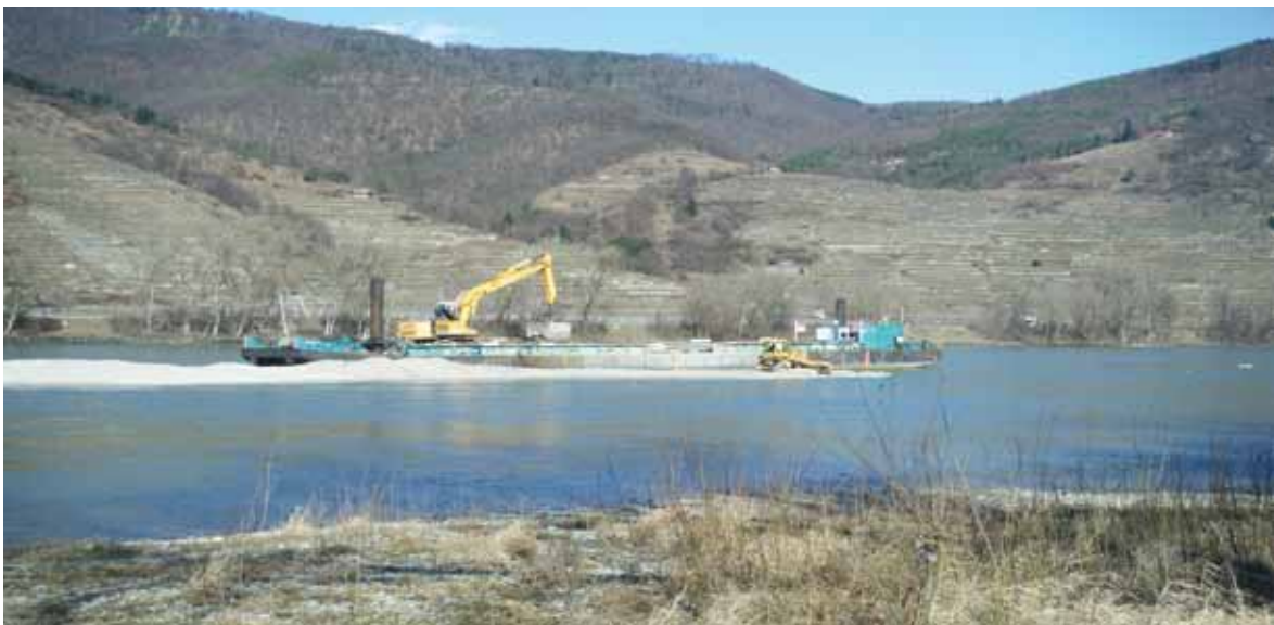
Dredging works with backhoe dredger in combination with hopper barges on the free-flowing section of the Wachau valley on the Austrian Danube; the excavated material is used to create new gravel islands in the river
