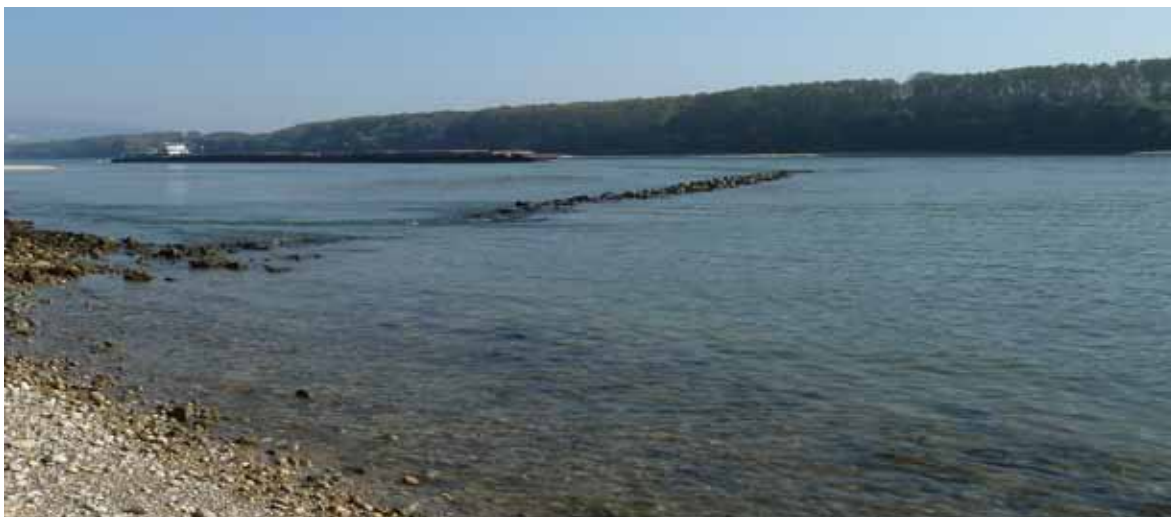
Declining groyne, i.e. adjusted to the river’s flow direction, for river regulation at low water levels
