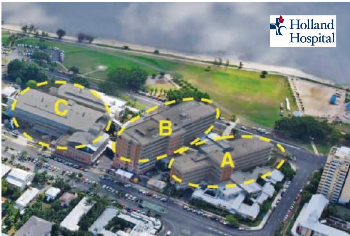
Figure 2: Holland Hospital plan with buildings A, B and C, esplanade and garden.
